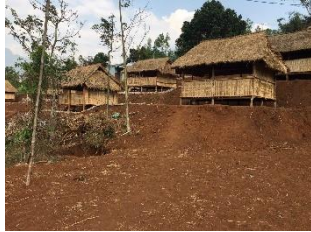
We built six huts to be used as classrooms
