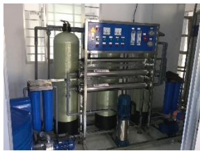
We built three water systems to provide clean water
